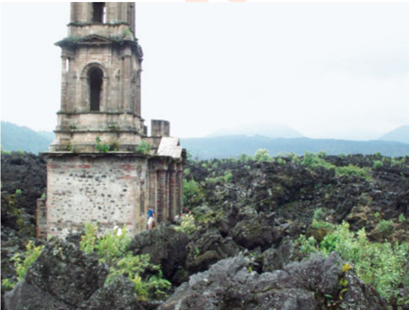
Fig. 2. Pahoehoe lava flows from Parícutín volcano broken into blocks and collapsing around the partly buried tower of the village church of San Juan Parangaricutiro. – Photo: B. Joyce, November 2003.
